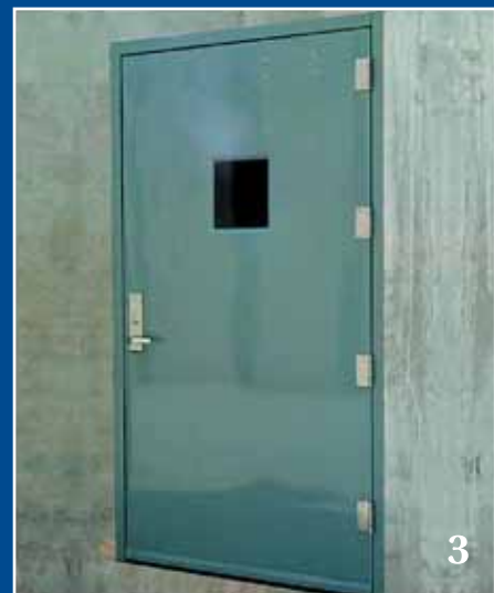
(3) Remove Straps – install anchors
